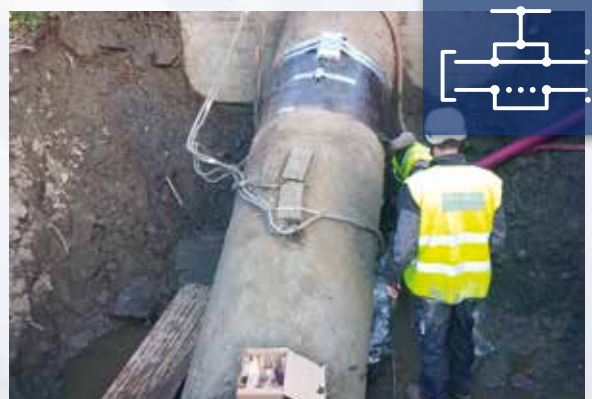
Installation of optical sensors for monitoring stress in a hydraulic pipeline
