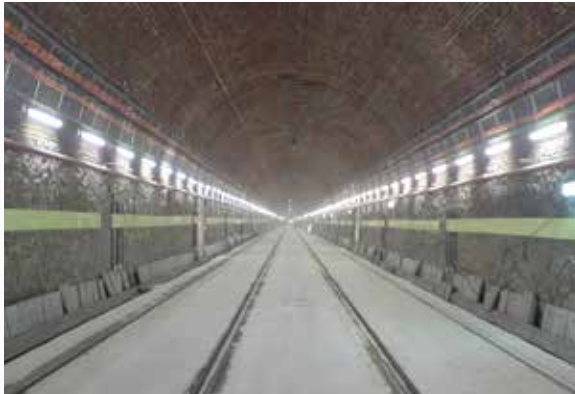
Instrumented cross-sections along the tunnel
