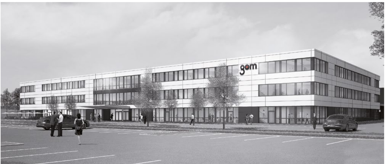
GOM headquarters in Braunschweig, Germany
