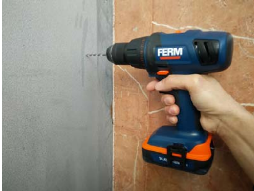
Fig. 2.4 Drilling the fixation holes
