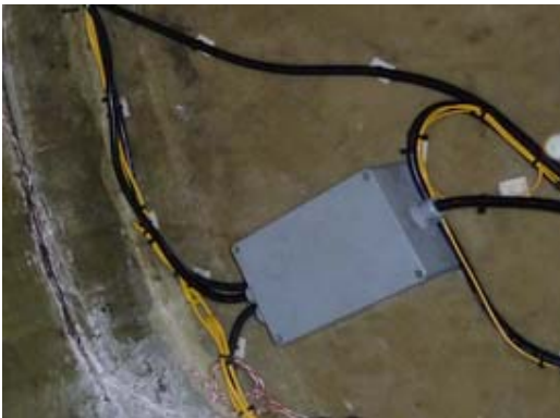
Fig. 2.9 Protection boxes for extra cable and connections
