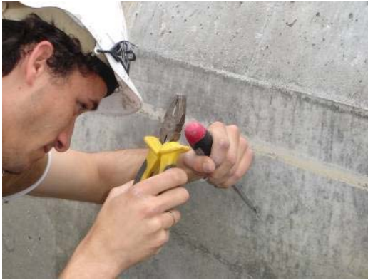
Fig. 2.1 Removing irregularities from the surface
