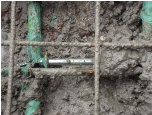
Fig. 2.13 Sensor during concreting
