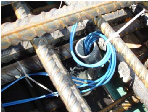
Fig. 2.2 Cable routing detail
