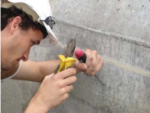
Fig. 3.1 Regularizing the surface
