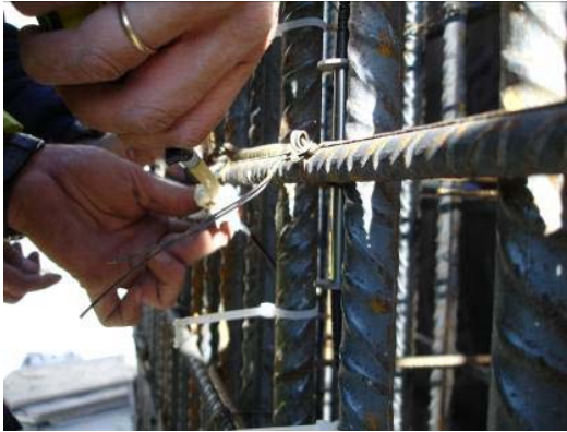
Fig. 2.12 Protection tube sealing
