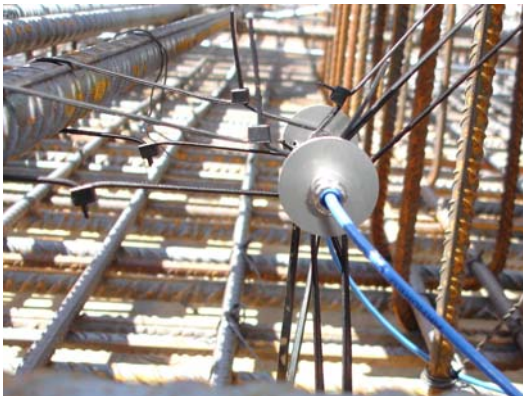
Fig. 2.8 Sensor's positioning
