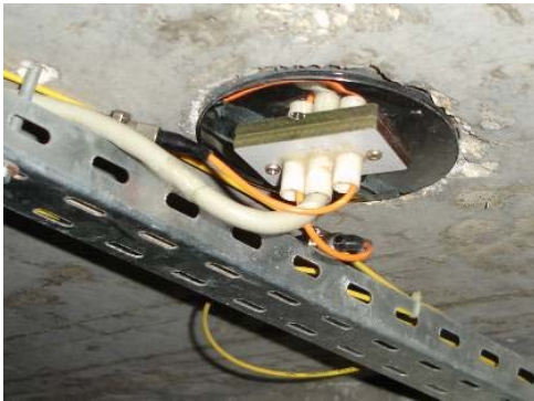
Fig. 2.6 Example of an embedded protection box
